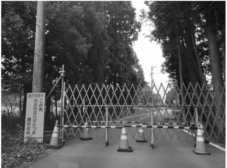
7. Damage caused by the Great East Japan Earthquake and Tsunami Disaster (Minamisanriku Town, Miyagi Prefecture).
