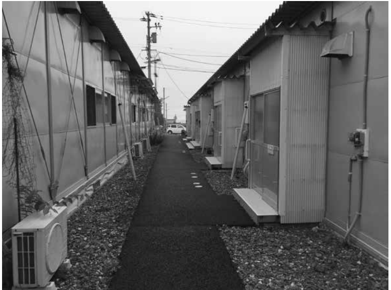
3, 4. Example of temporary emergency housing (3. Koriyama, Fukushima Prefecture; 4. Otsuchi Town, Iwate Prefecture).
