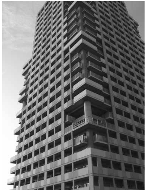
6. Example of disaster public housing after the Great Hanshin and Awaji Earthquake (Kobe City, Hyogo Prefecture).
